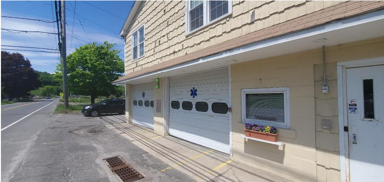
In addition, modifications must be made to ambulances after purchase to allow them to be stored in such a small space. Vehicles have struck the building twice. In addition, the apparatus bay floor is below grade from the road resulting in drainage issues with water intrusion during wet weather events.
